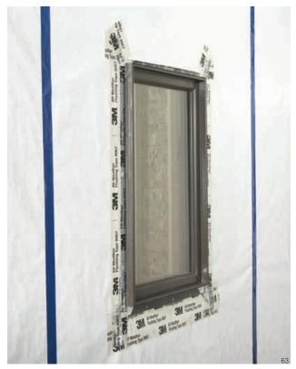
$3M^{\rm \tiny TM}$  All Weather Flashing Tape 8067 is a self-adhered, waterproof flashing membrane designed for sealing around openings and penetrations in exterior walls.
