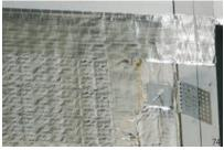
3M<sup>™</sup> FSK Facing Tape 3320 is engineered specifically as a vapor retardant tape to seal mineral wool foil-faced insulation, bare sheet metal ducts and blanket style fiberglass duct insulation.
