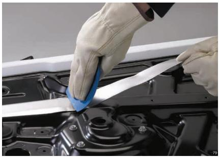
Applied with a 3M<sup>™</sup> PA-1 Wiper to the inside of a car door, 3M<sup>™</sup> Damping Foil 2552 effectively damps noise and vibration with as little as 10% surface coverage. Optimized acrylic on a dead soft aluminum constraining layer converts vibrational energy to negligible heat that readily dissipates.
