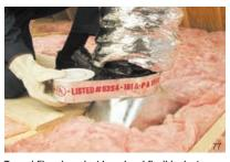
To seal fiberglass duct board and flexible duct systems, Scotch® Foil Tape 3326 meets the performance requirements for UL 181A-P and UL 181B-FX.
