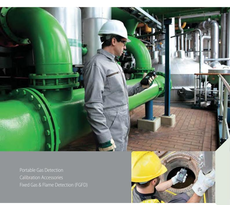
Battery-powered, direct-reading portable instruments are classified into two groups - single-gas instruments or multiple-gas instruments. Depending on the capabilities of the instrument, monitoring can be conducted simultaneously for oxygen and combustible gas, or for oxygen, combustible gas and toxic gases. These devices are commonly referred to as 2-in-1, 3-in-1, 4-in-1 or 5-in-1 alarms.
