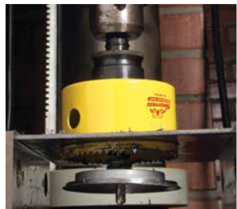
After the hole has been drilled, the core can clearly be seen at the end of the pilot drill.
